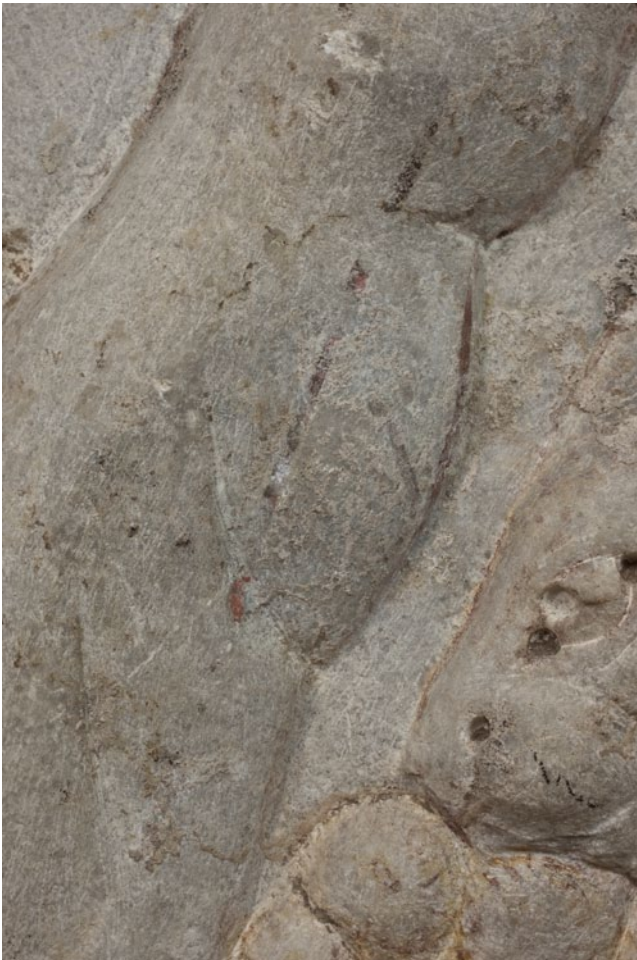
Fig. 15: Detail photo of the right leg of the centre cupid. The removal of secondary mortar on top of the painted dark lines reveals the beautiful red colour of cinnabar underneath.
